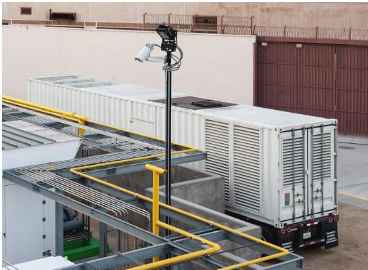
Figure 22: Backup mobile diesel generator at LA Metro Division 13, Los Angeles, CA.
