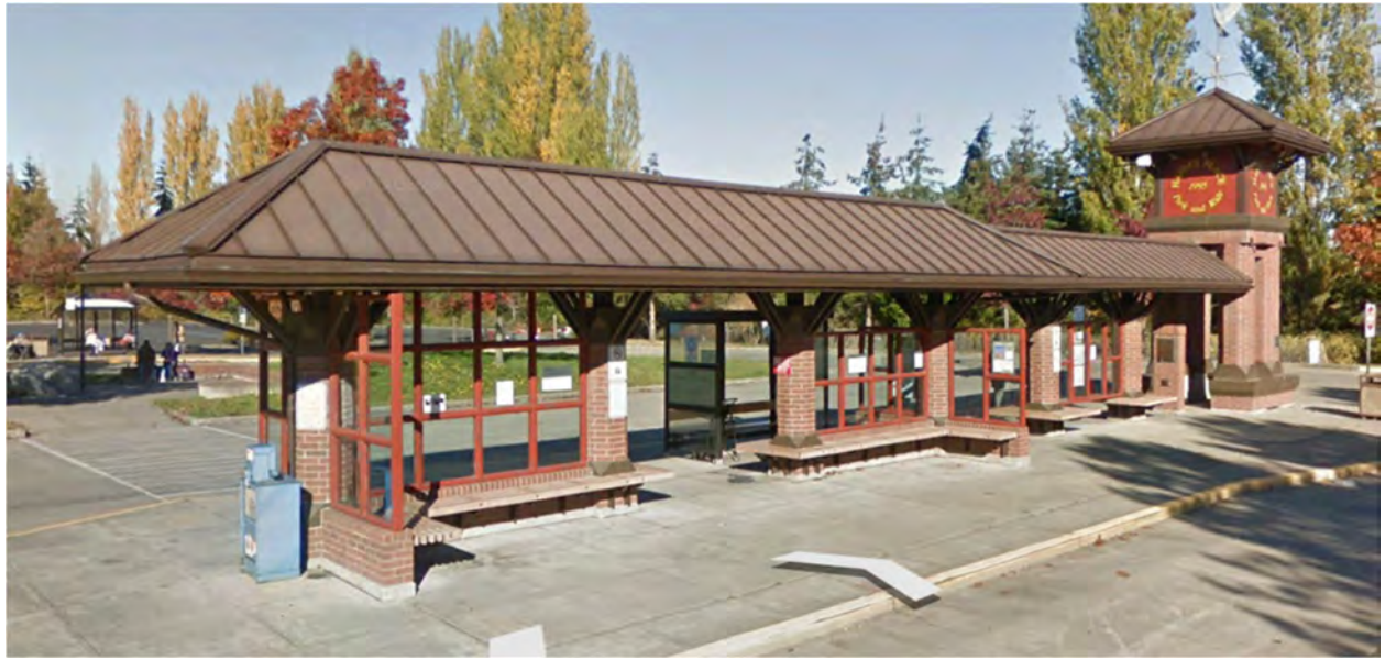
Figure 14: Purpose-Built Shade/Wind Structure in Port Townsend, Washington
